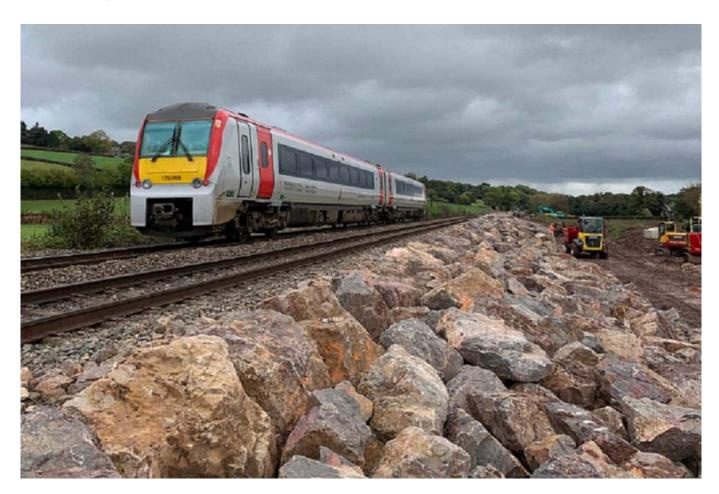
As part of a project to protect the network running between Hereford and Abergavenny, engineers have installed 8,000 tonnes of 'rock armour' to fend off the elements.
