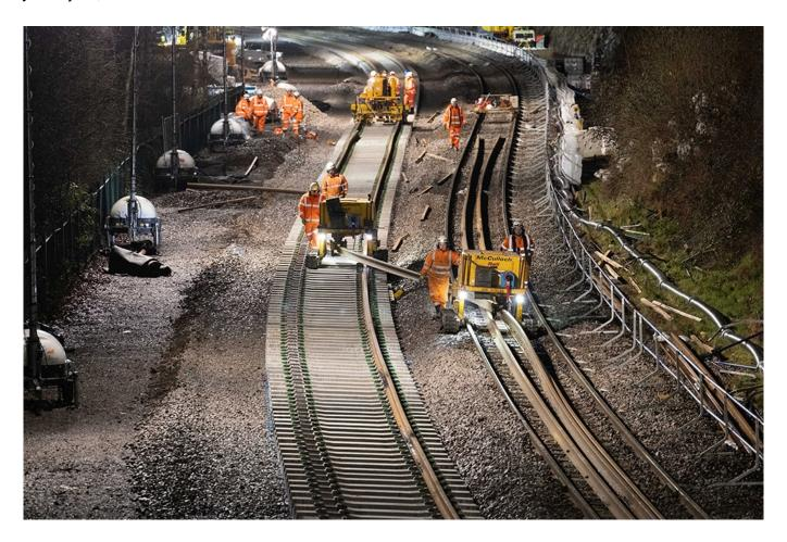
Work to transform Morley station continues later on this month with Network Rail laying the foundations for new, longer platforms, realign the track to support faster trains through the area and complete important drainage work.
