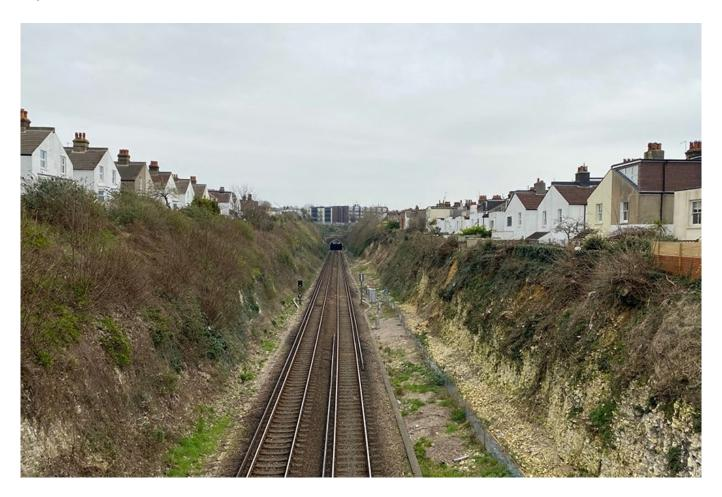
Engineers are preparing to improve and strengthen a section of track at Hove between Saturday 18 September 2021 and Friday 1 October 2021. These works are planned to stabilise a section of railway cutting in Hove and prevent landslips, which have caused significant delays to passengers in recent years.
