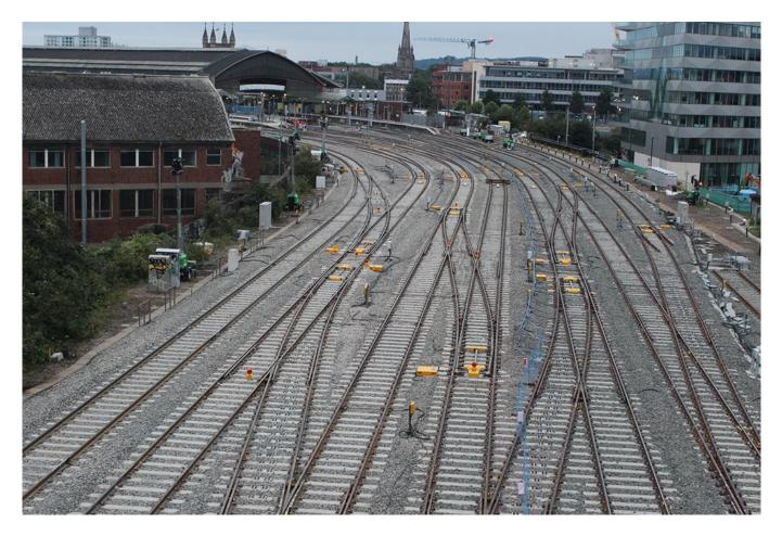
Network Rail has completed its major upgrade of Bristol East Junction, removing a bottleneck into Bristol Temple Meads and replacing the 1960s track and components. This will allow more trains to enter and exit the station, increase capacity, reduce congestion and help make journeys more reliable.
