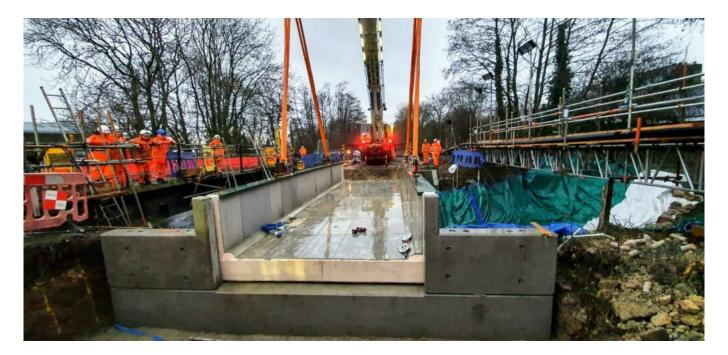
Engineers have worked around the clock over the last four days to replace the deck of a 129-year-old bridge, as part of a series of improvements on the Heart of Wessex line between Weymouth and Yeovil Pen Mill.
