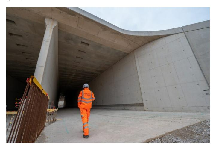
HS2's main works civils contractor in the West Midlands, Balfour Beatty VINCI (BBV), has completed the construction of the 200 metre porous portal of HS2's Burton Green Tunnel.
