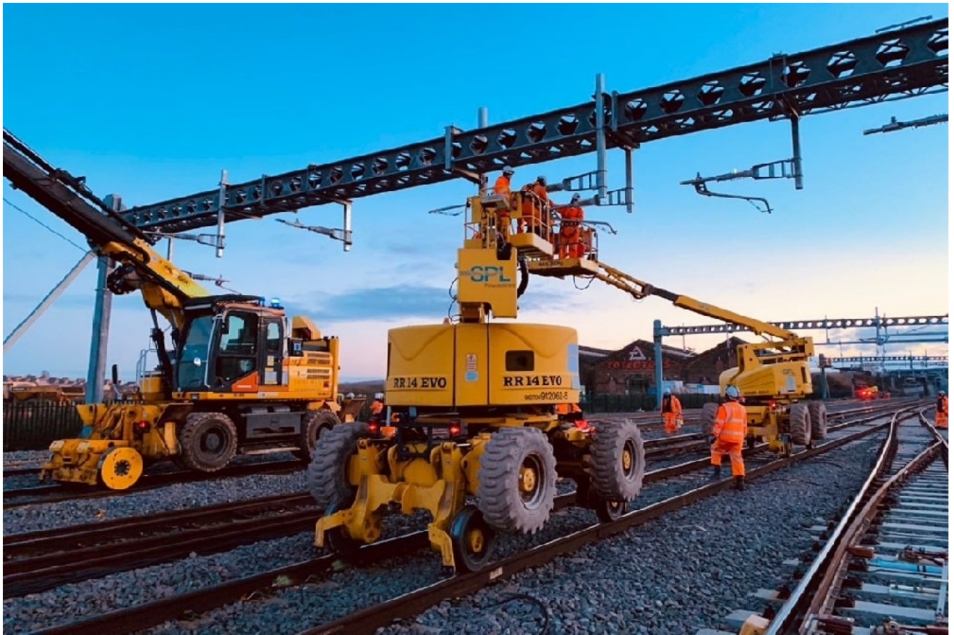
Previous overhead line equipment already in place
