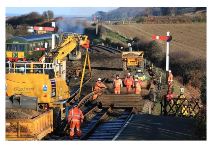
New pointwork costing over £300,000 is being installed at the eastern end of Weybourne Station on the North Norfolk Railway.
