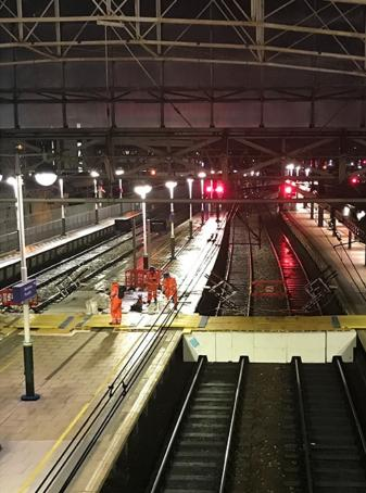
Polystyrene blocks have been used by Network Rail to bridge the gaps between platforms to build a temporary route along the width of Manchester Piccadilly railway station so that mobile elevated working platforms (MEWPs) could reach the roof structure.
