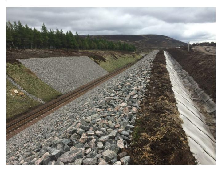
Work is underway on a final phase of embankment and drainage work at Slochd between Perth and Inverness on the Highland Mainline.
