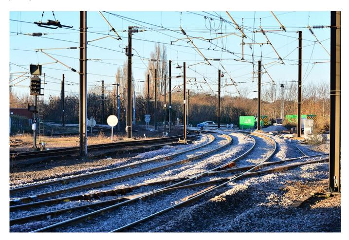
Network Rail has refreshed nearly 3km of track through the platforms at York railway station. The £6 million upgrade will help to drive down delays, getting passengers where they need to be on time, and improve the track's condition for many years to come.
