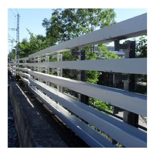
Even in the most difficult situations the Elevated Troughing System can be adapted to work. Rock-based terrain where the application of mounting pillars could create extensive additional work. Here the product is adapted to the natural rock through the cutting providing a safe cable management trough which can be easily maintained.
