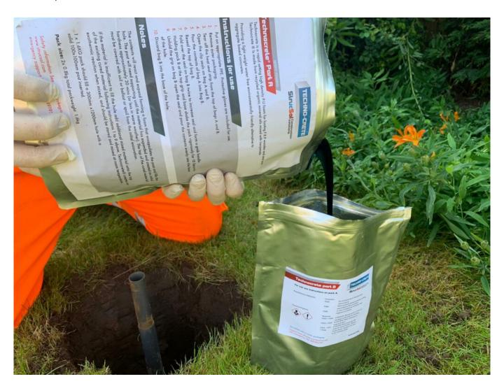
Network Rail-approved supplier Scott Parnell's Techno-Crete is a new innovative alternative to postmix concrete used for securing fence posts, gates, elevated troughing, sign posts and marker boards.
