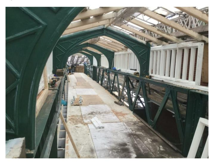
Work to upgrade Shrewsbury station continues with repairs and the renewal of station canopies almost complete and work progressing on the refurbishment of Dana footbridge.
