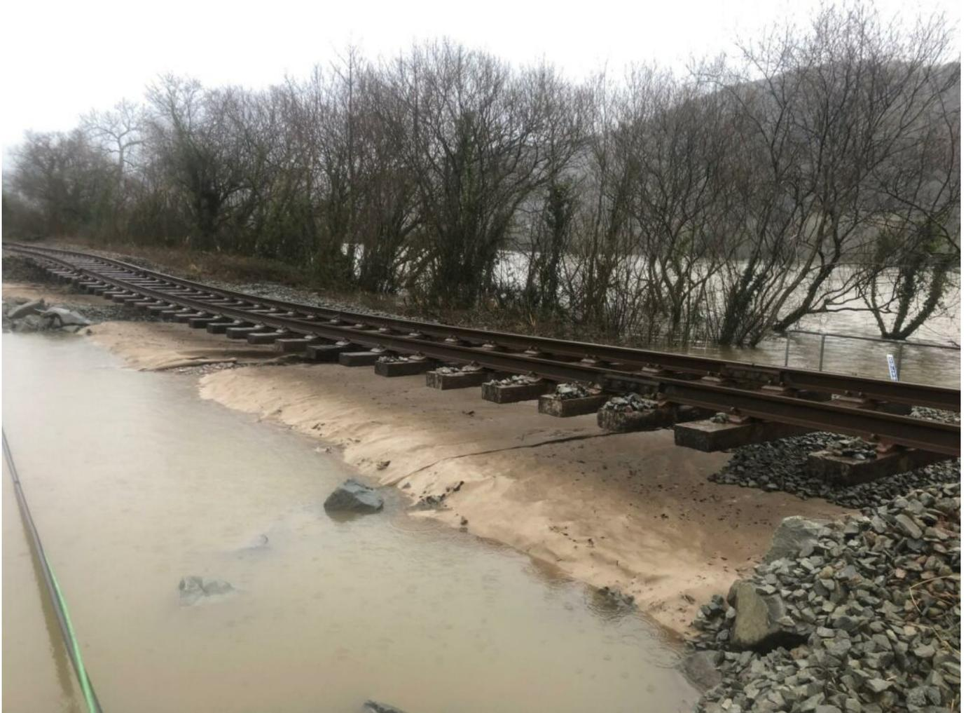
Storm Ciara, which brought 90mph winds, extreme rainfall, and flooding across Wales, has caused extensive damage on the Conwy Valley Line, north of Llanrwst.
