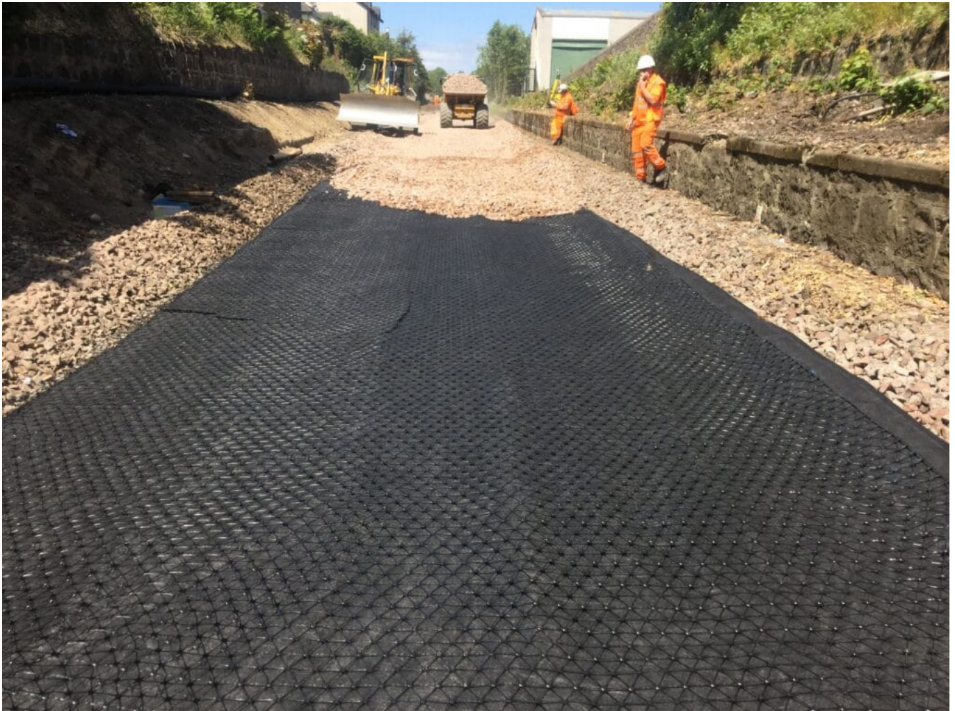
Mechanical stabilisation of track ballast and sub-ballast with Tensar geogrids
