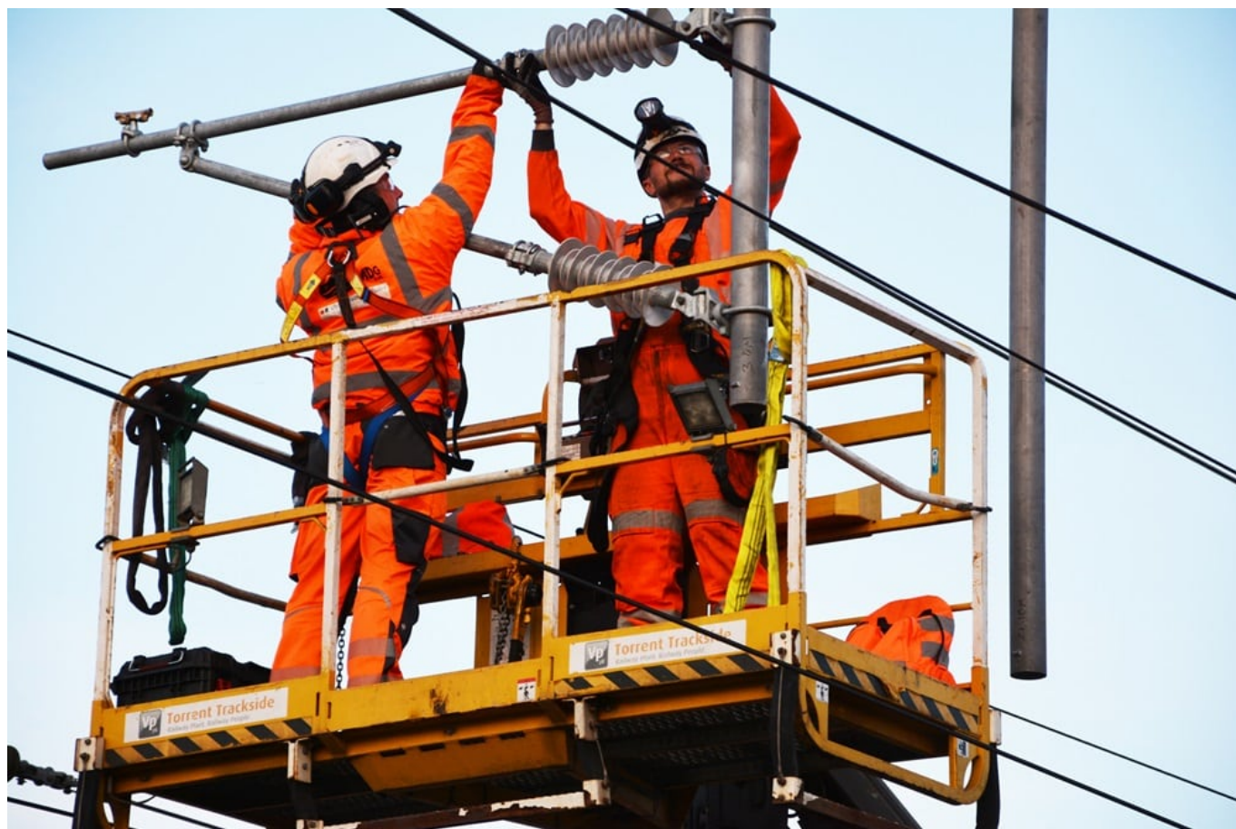
The machines provide a spacious and stable platform for OLE work. Credit: Torrent Trackside.
