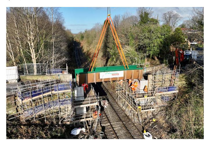
Network Rail has made major progress on the Transpennine Route Upgrade in Manchester after raising two railway bridges to make way for overhead electric wires.
