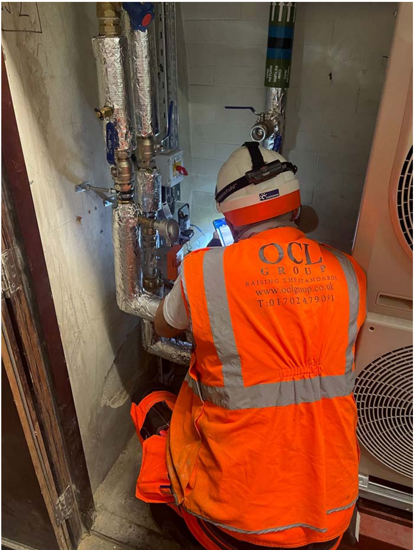
The OCL team at work on the project
