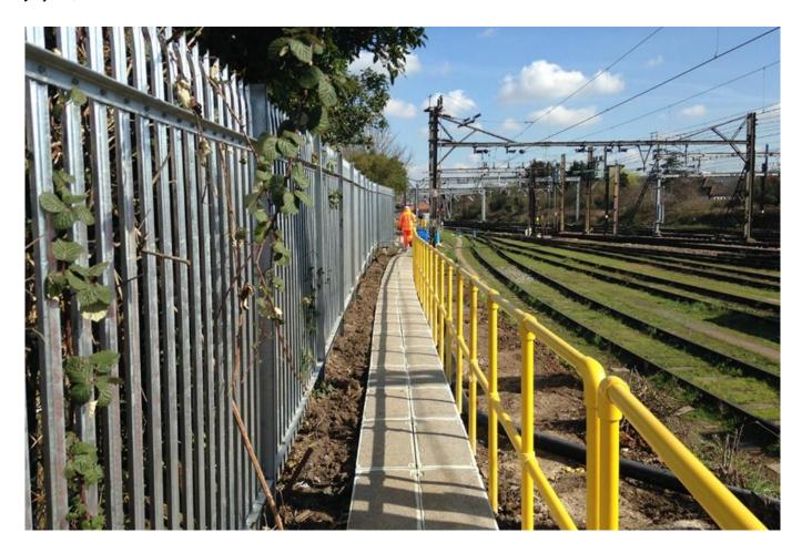
The TTS Walkway system is designed to provide a hard wearing and safe surface for troughing routes where a low to zero maintenance walkway is required.
