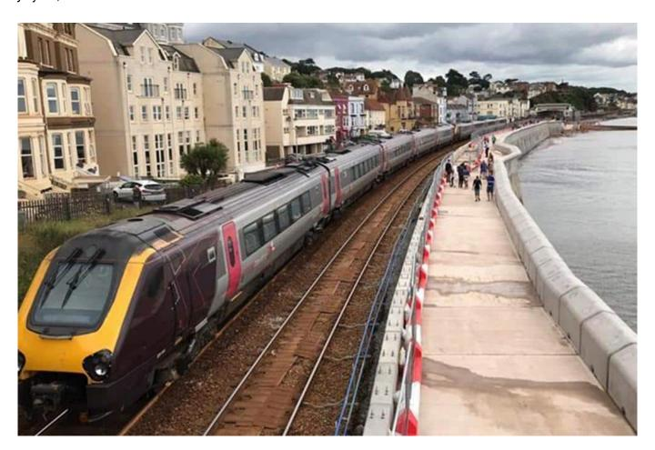
The vital stretch of railway which connects Devon and Cornwall with the rest of the country is now better protected from rising sea levels and extreme weather as Network Rail has built the first section of the new sea wall in Dawlish.
