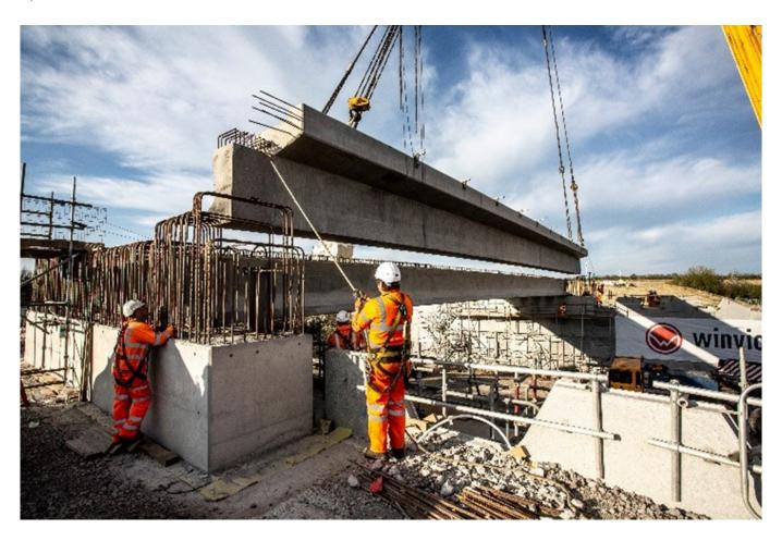
Winvic Construction Ltd, a leading main contractor that specialises in the design and delivery of multisector construction and civil engineering projects, successfully lifted eight railway bridge beams into place over the A5 – 2km north of M1 J18. It is one of three bridges that Winvic is constructing for Prologis at DIRFT III in Northamptonshire, as part of a £29 million contract to deliver a new state-of-the art Intermodal Rail Freight Terminal.
