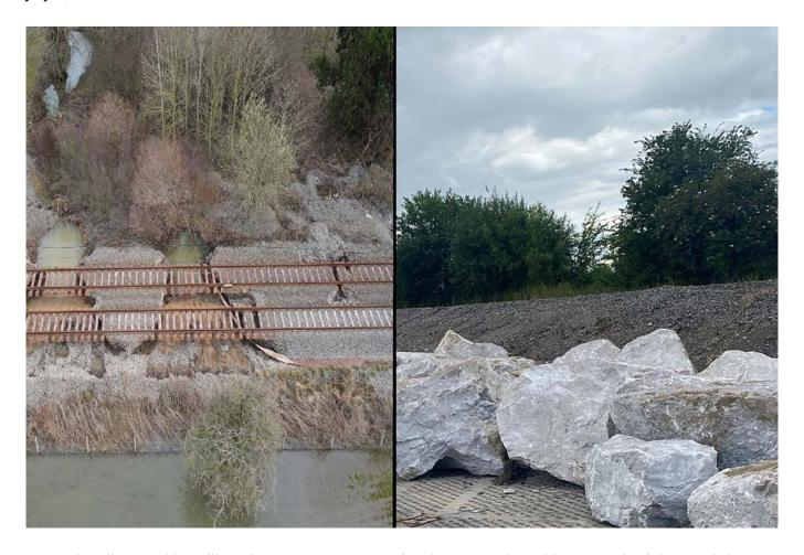
Network Rail started installing about 10,000 tonnes of rock armour alongside a stretch of the Cambrian Line to make it more resilient.
