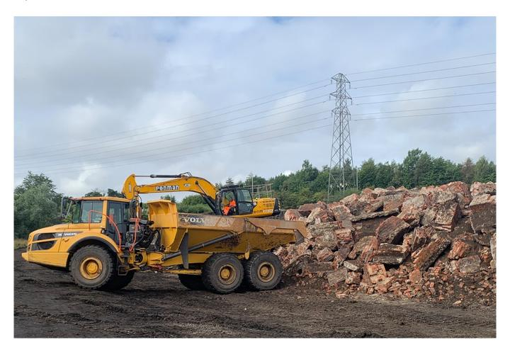
Platform removal has cleared the way for double tracking at Cameron Bridge.
