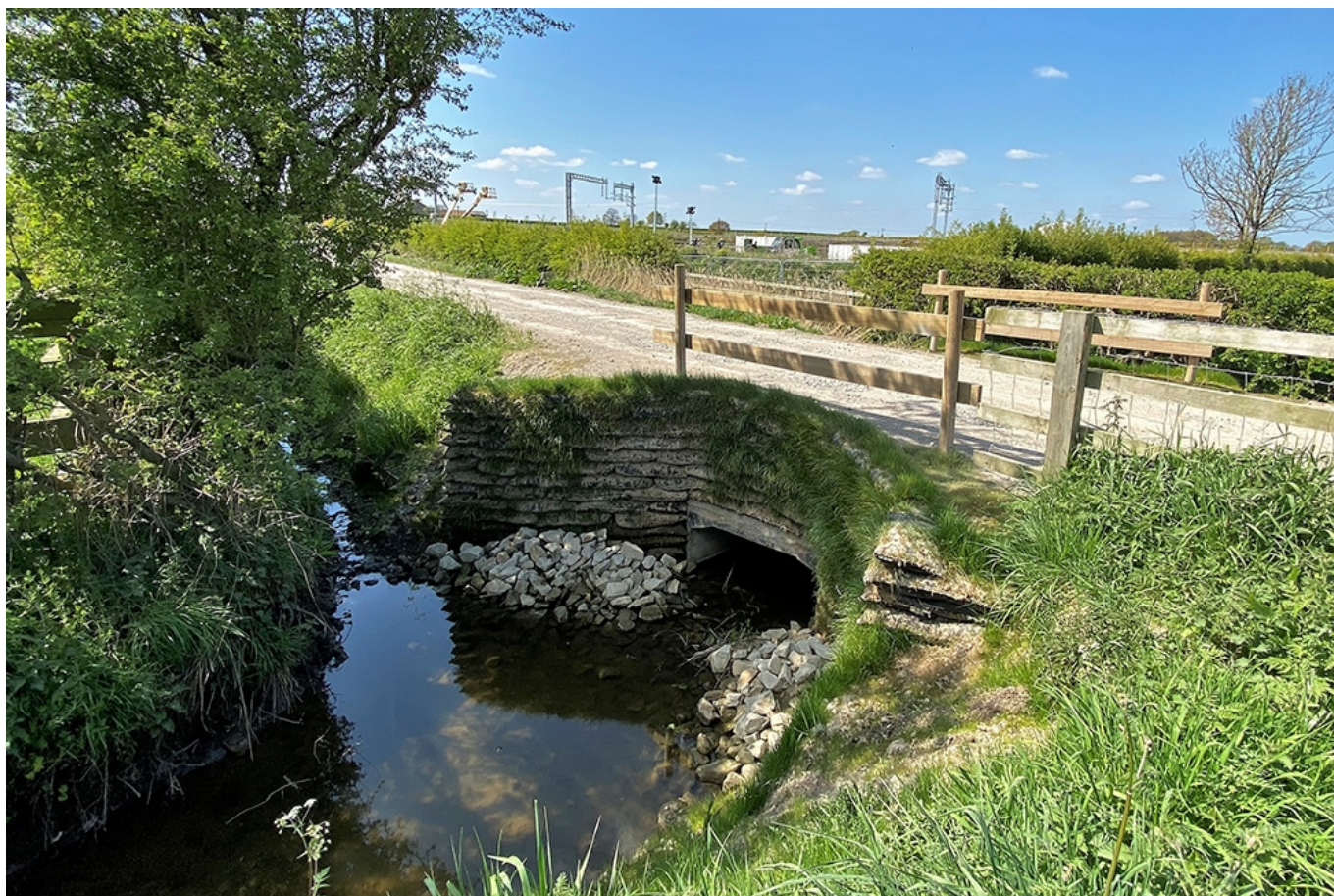
Flex MSE vegetated culvert headwall
